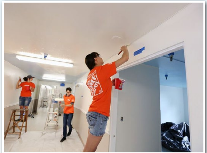
Home Depot volunteers work on interior.
