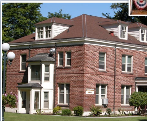
The Betsy Ross Building in Orting, WA
